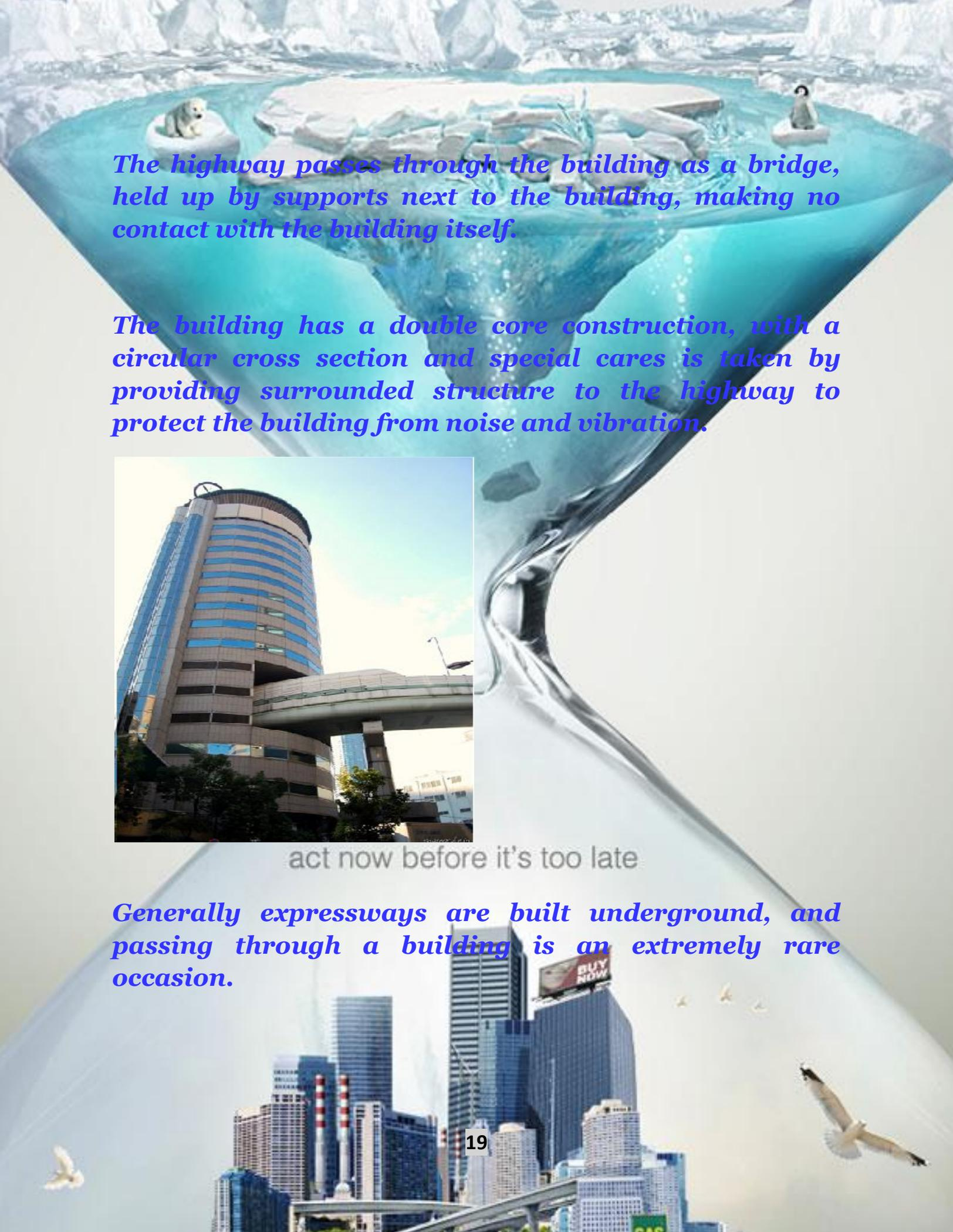
*The highway passes through the building as a bridge, held up by supports next to the building, making no contact with the building itself.*
